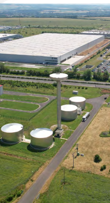
Water tower with drinking water and water tanks with filtered river water / vodojem s pitnou vodou a zásobníky průmyslové vody
